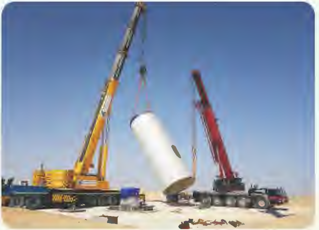
Example of a WTG being installed onto a concrete foundation with crane
