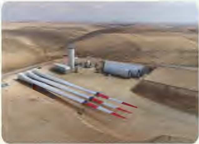
Example of WTG components including tower, blades, nacelle and hub
