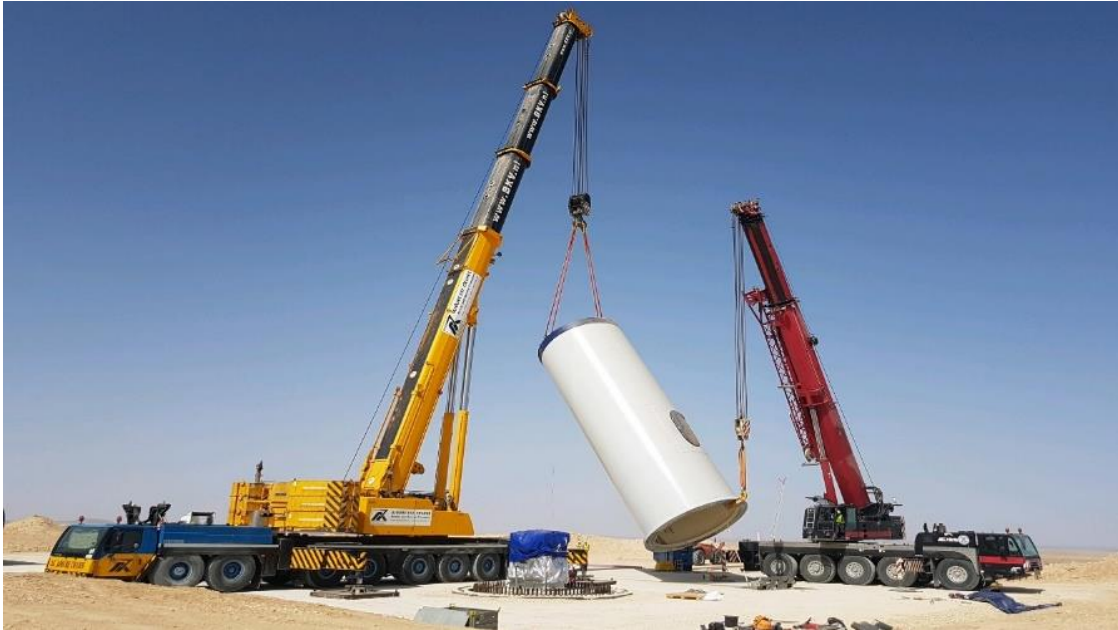
Figure 2.3: Example of WTG erection and installation
