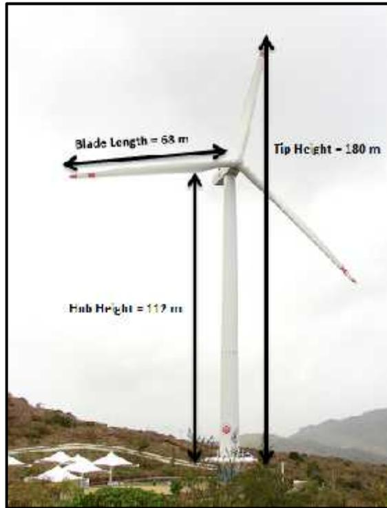
Figure 2: Typical Wind Turbine with 180m Tip Height
